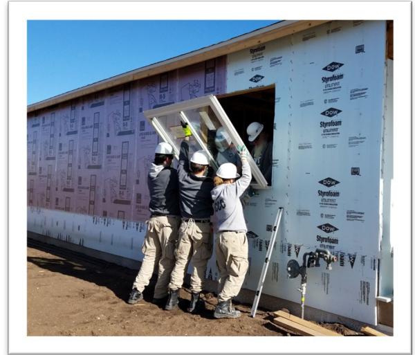
AmeriCorps NCCC Team installing a window on the 2nd Annual Veteran Home Build
