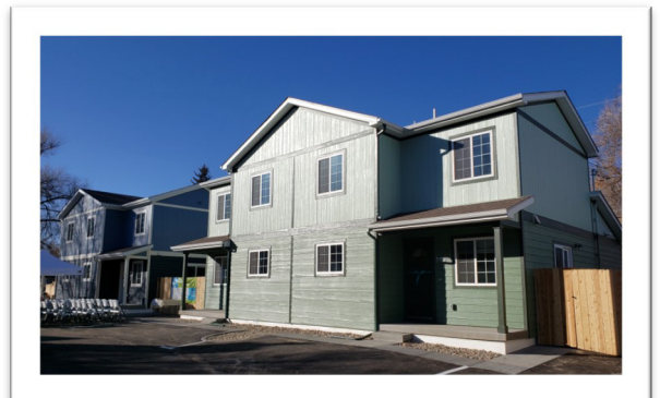
The four homes of Little Village Subdivision on Dale Street in Colorado Springs
