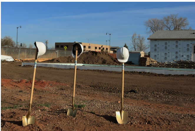
Preparation for the 2020 Thrivent Faith Build Ground Blessing in Fountain, CO.
