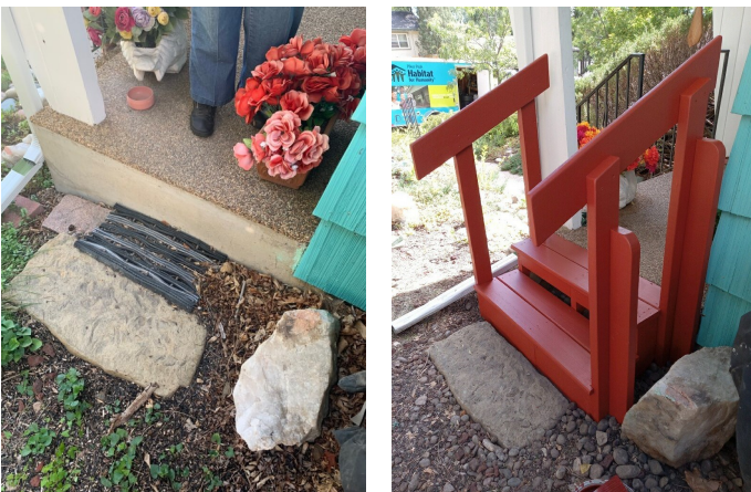
This homeowner’s porch posed a falling hazard, so the repair crew added steps and railings.
